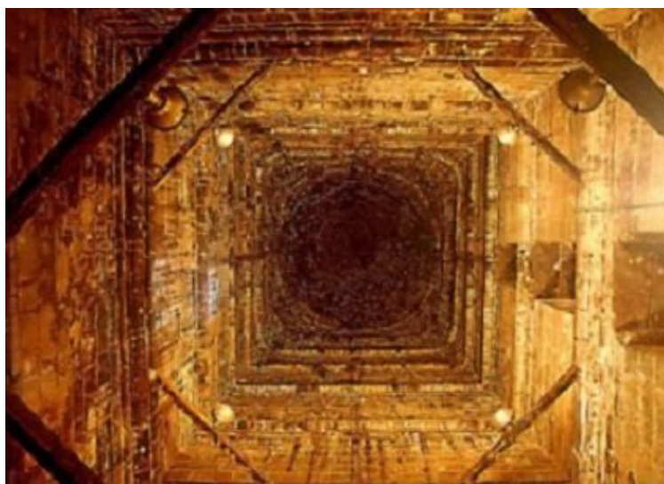
The hollow interior of the Thanjavur Viman Temple, a view from below, right from Garbha Griha HariBhakt
